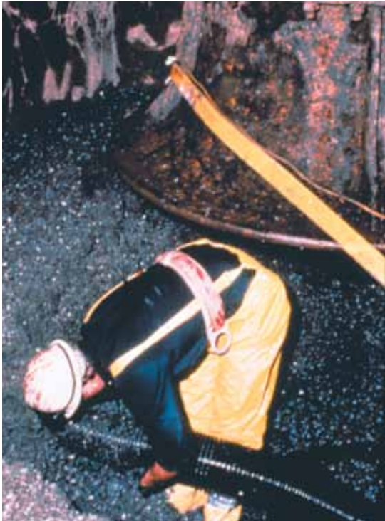
A worker uses a hose to suction zebra mussels from inside a pipe at a power plant.
